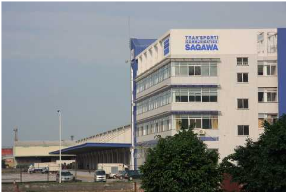
Shekou Logistics Center
